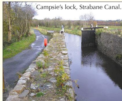
The locks were designed to accommodate sea-going schooners, capable of carrying 300 tons of cargo. Devlin's lock was 108ft by 23ft (33m by 7m), with 7ft (2.1m) of water over the cill, while Campsie's Lock was 117ft by 24ft (36m by 7.3m), with a depth of 6.5ft (2m). Tolls were collected by the Marquess's agents at a flat rate of two shillings (10p) per ton. Lighters were towed by a steam tug to the entrance of the canal, while horses provided the power for the journey up to Strabane.
