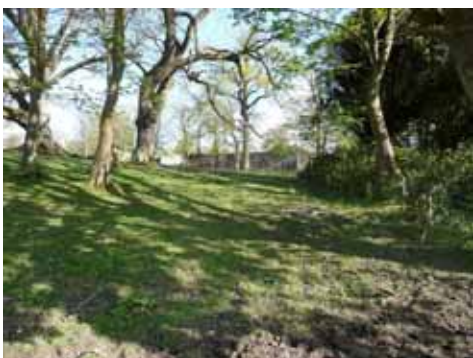
Boom Hall Stable Building
