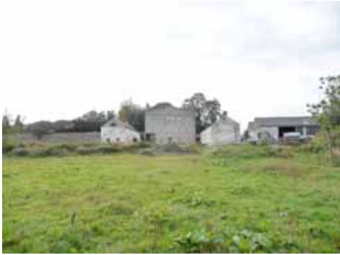
Port Hall, former Port side
