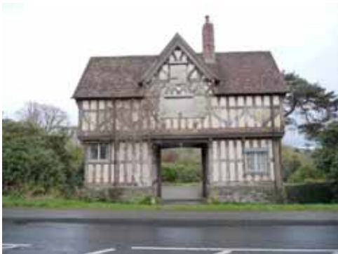
Sion House gatelodge, Sion Mills
