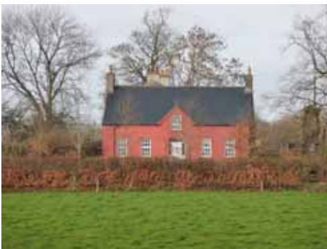
Longvale House, Porthall
