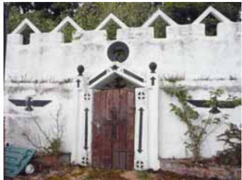
Ravenscliff, Moville; WW2 section of garden wall
