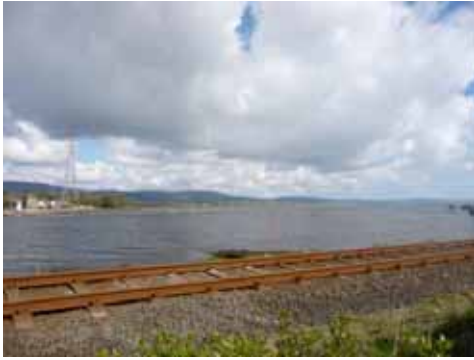
Railway & Culmore point at narrows into the lough
