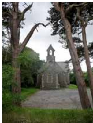
St Finian's, Redcastle; designed by Welland & Gillespie
