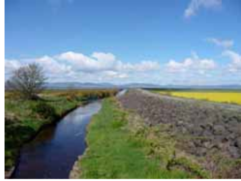
Broharris Canal/ Ballykelly river
