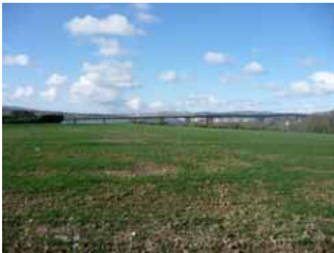
Gransha view to Foyle Bridge & city to the south
