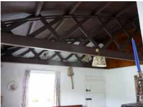
The "Onion Baskets" Belfast roof structure
