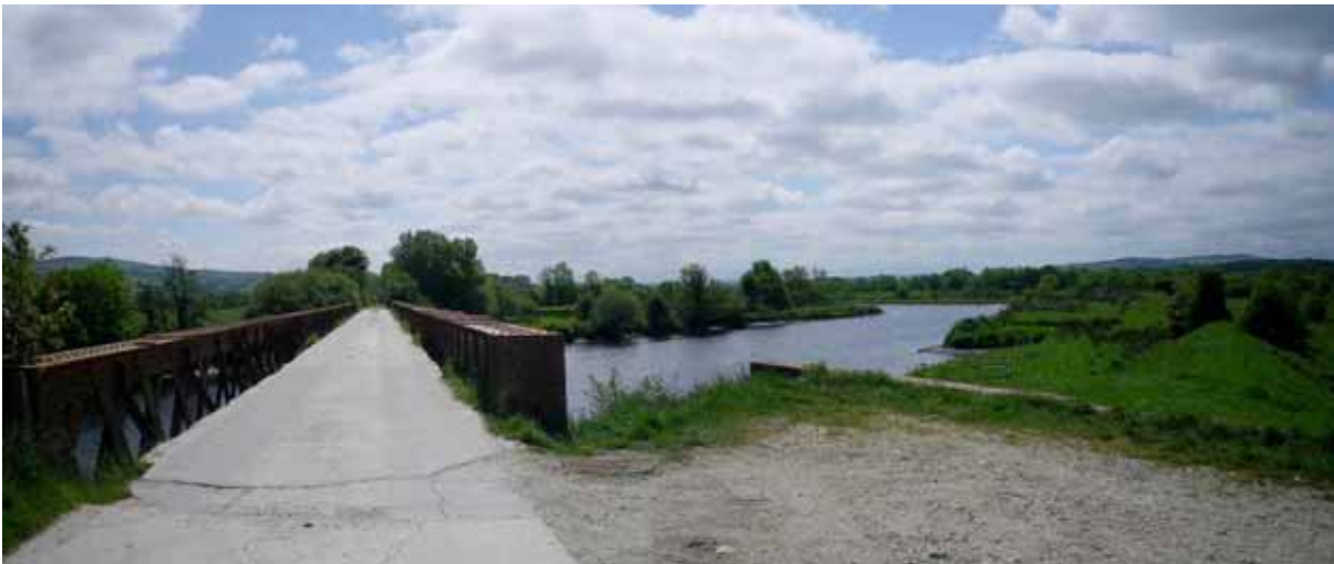
Corkan Isle trestle bridge
