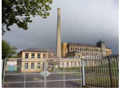
Herdman's mill after damage by fire, Sion Mills
