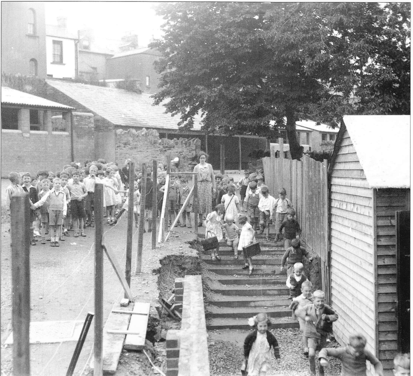
Here the children from the Model School are keen to get home or to class, not minding the building work. Nicholson Terrace can be seen in the background. (SCH 2-12)
