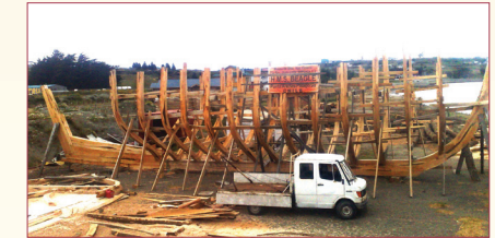
The construction of the HMS Beagle Full Size Replica by locals
