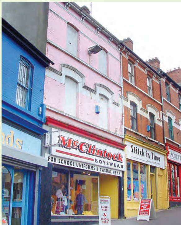
Prior to refurbishment
