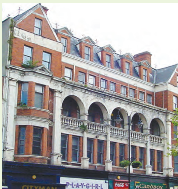
Prior to refurbishment
