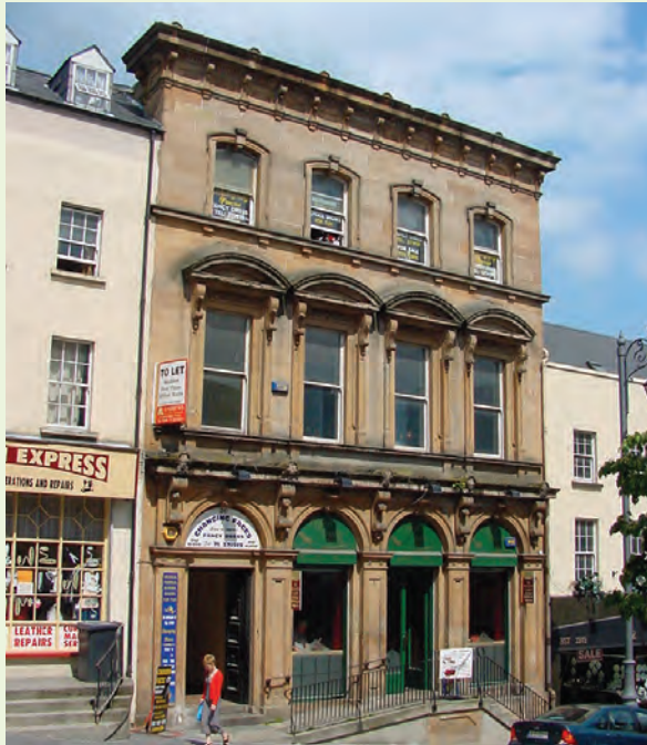
Prior to refurbishment
