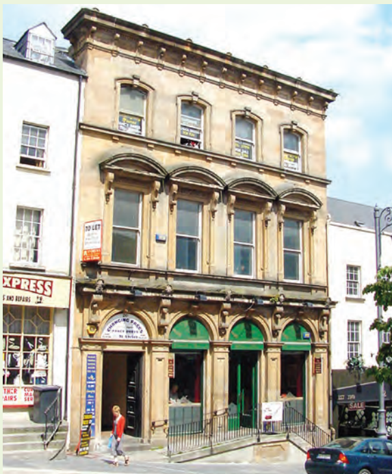
Prior to refurbishment
