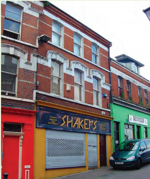
Prior to refurbishment
