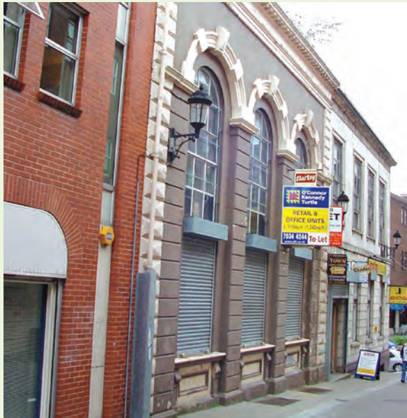
Prior to refurbishment
