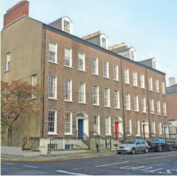
Nos. 13–16 Queen Street
