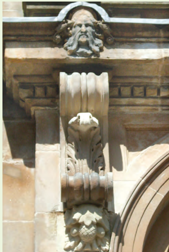
Restored moulding detail (new pineapple detail and acanthus leaf repair).
