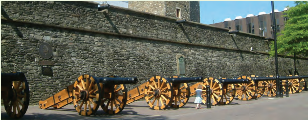
Shipquay Place with restored cannons in 2006.
