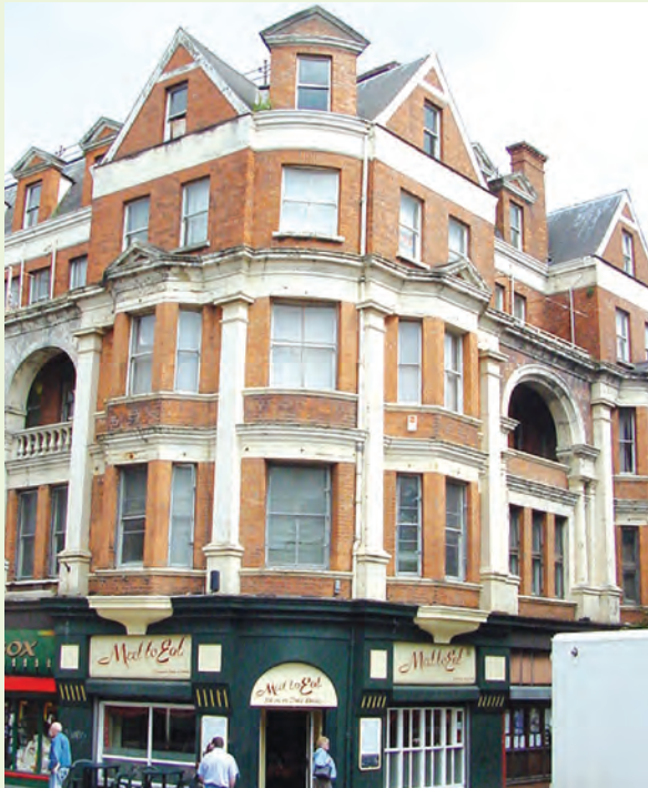
Prior to refurbishment
