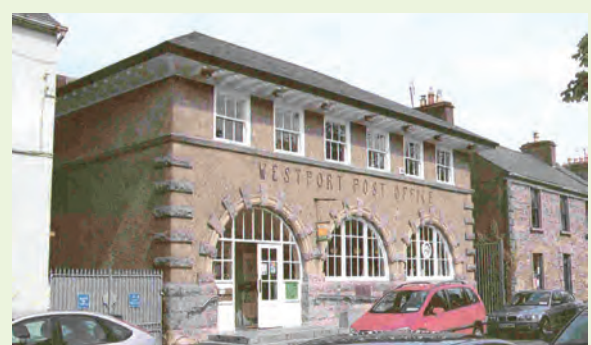
Post Office, North Mall
