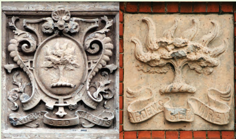
Verbal Arts Centre, external detail
