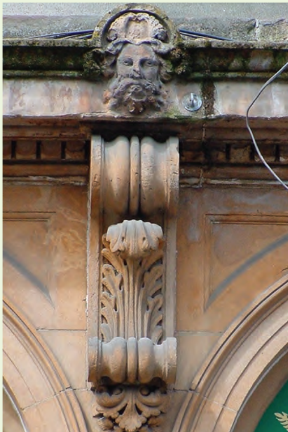
Existing moulding detail.
