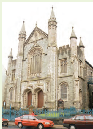
4th Derry Presbyterian Church, Carlisle Road
