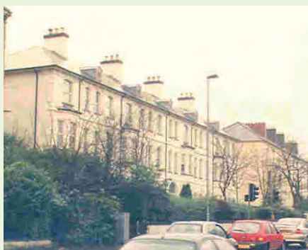
Replacement terrace of apartments on Northland Road.
