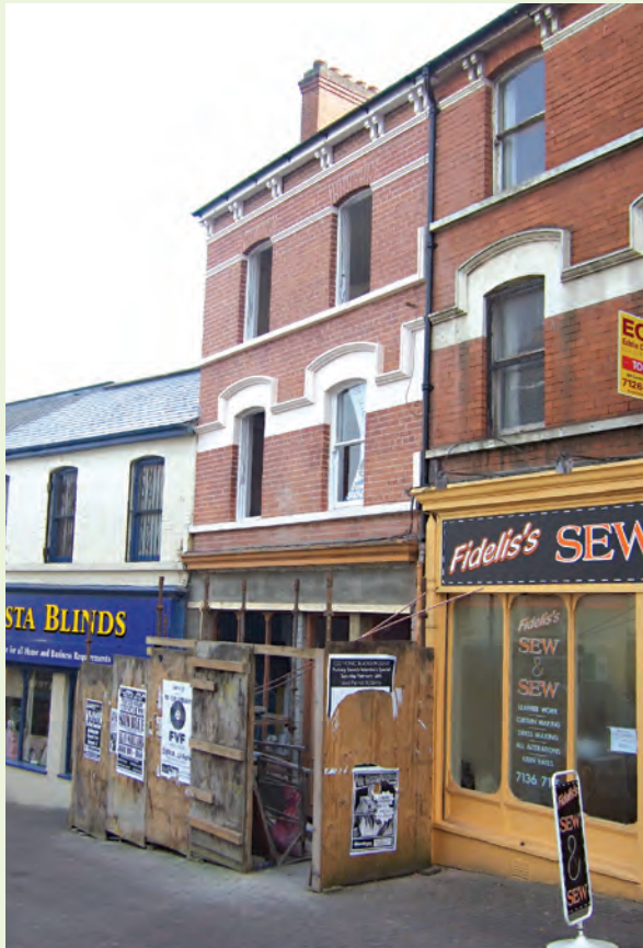
Prior to refurbishment
