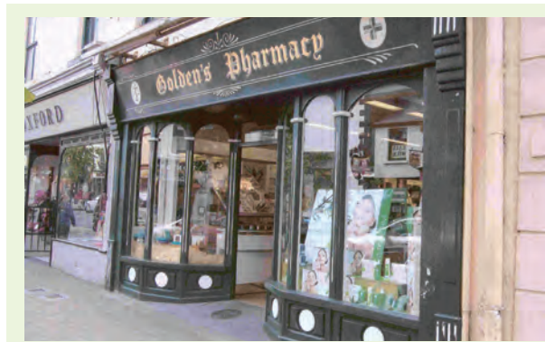
Shopfront, Shop Street
