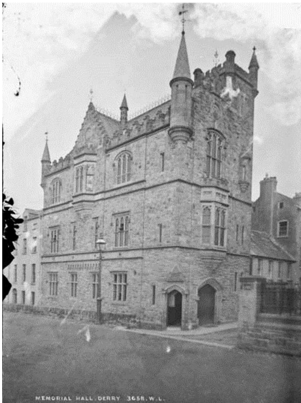
Apprentice Boys Hall, circa 1900 Hall has splayed corner entrance doorway at Upper Magazine Street and double doors to Society Street.
