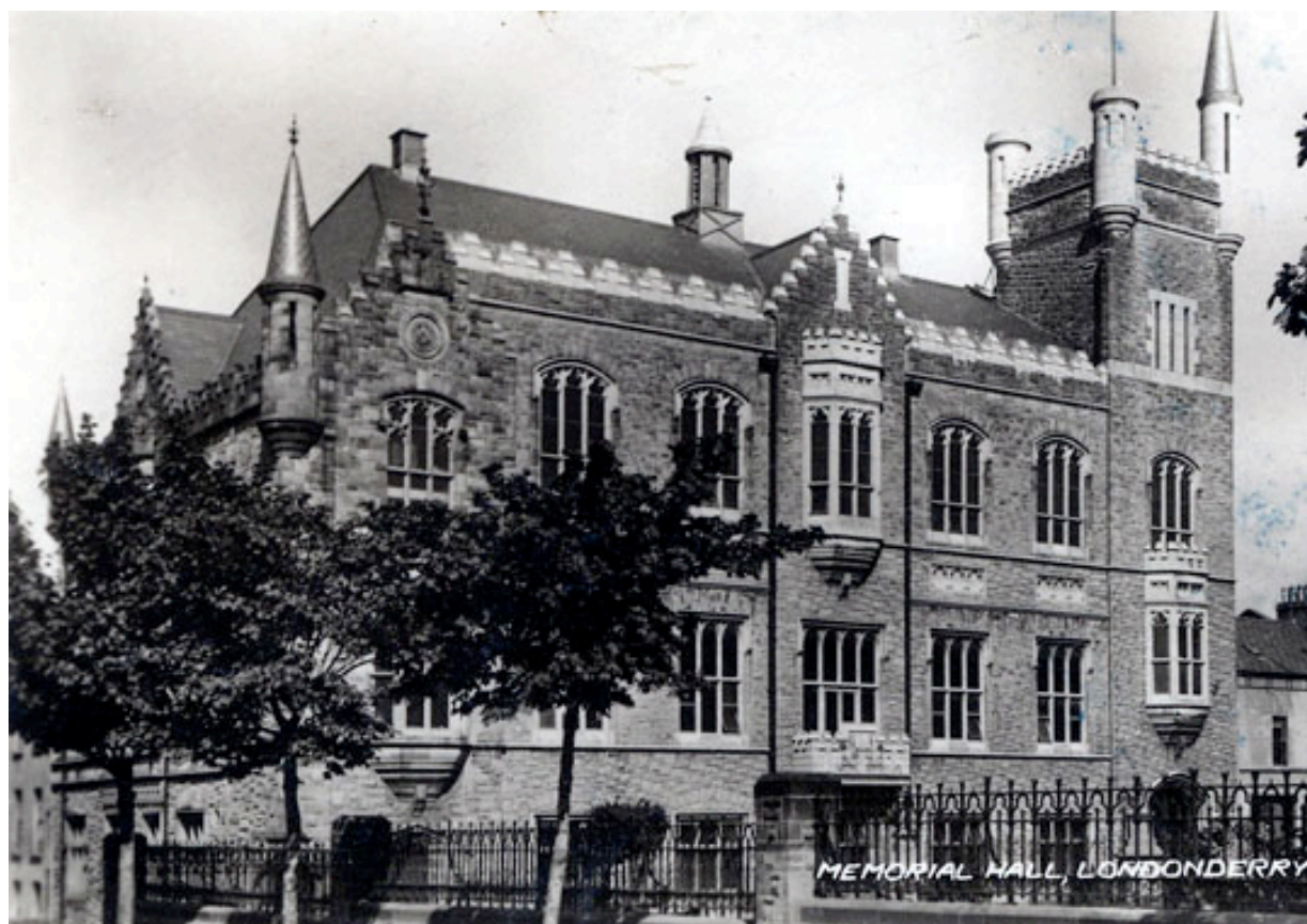
Apprentice Boys Hall extension completed, circa 1940
