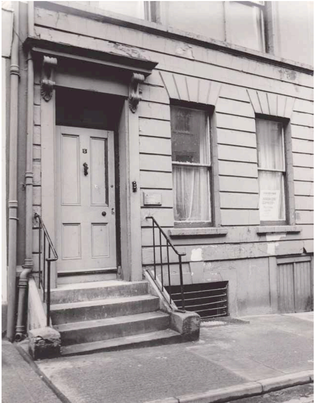
Door detail, 5 Pump Street, circa 1975
