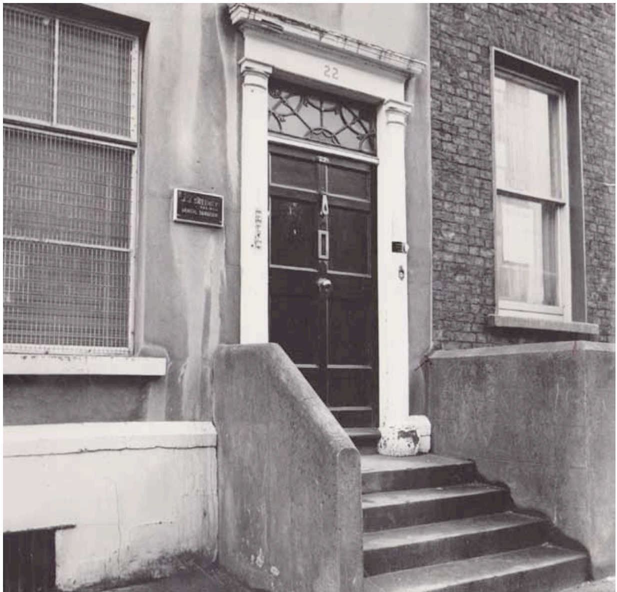
Door detail, 22 Pump Street, circa 1975
