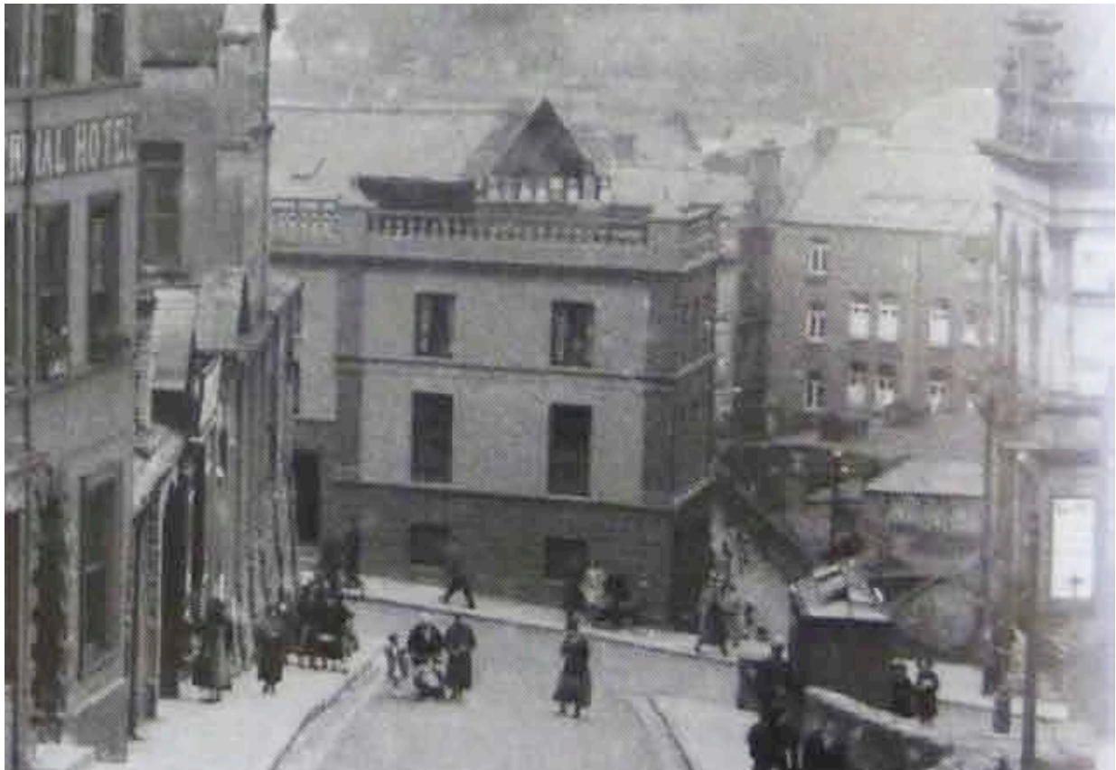
Newmarket Street elevation of 11 East Wall, viewed from Market Street, circa 1930
