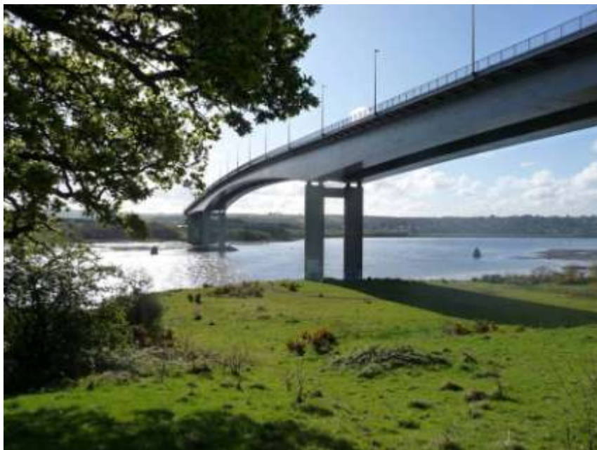
Figure 314 – Foyle Bridge constructed 1984; the longest bridge in Ireland
