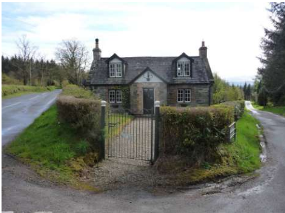
Figure 238 – Baronscourt estate buildings
