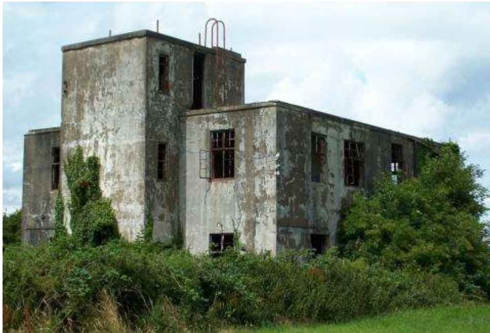
Figure 127 – Aghnaloo airfield tower (c) ww2ni.webs.com
