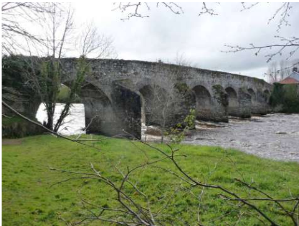
Figure 225 – Newtown Stewart Bridge
