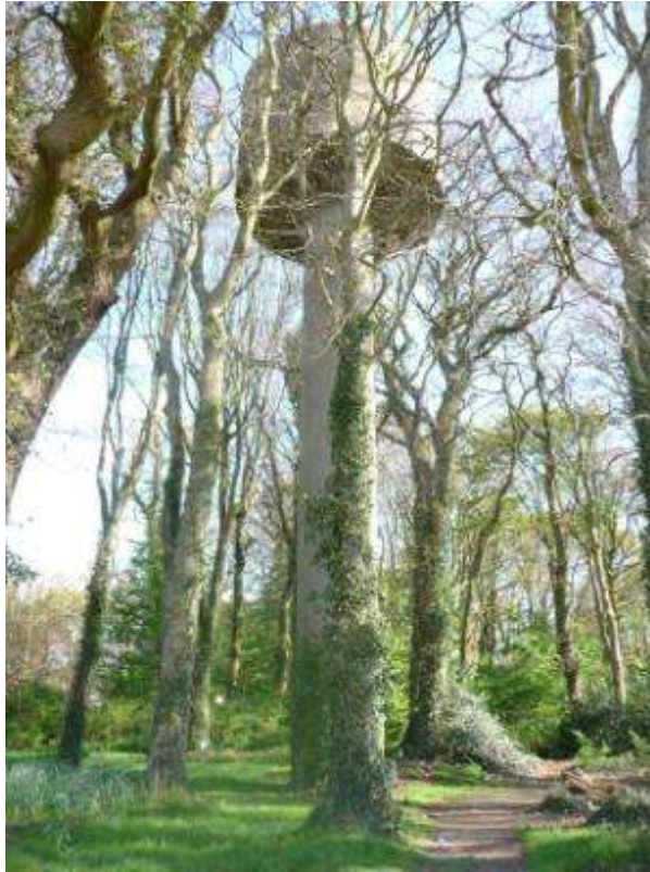
Figure 67 – Gransha Woods and concrete water tower.
