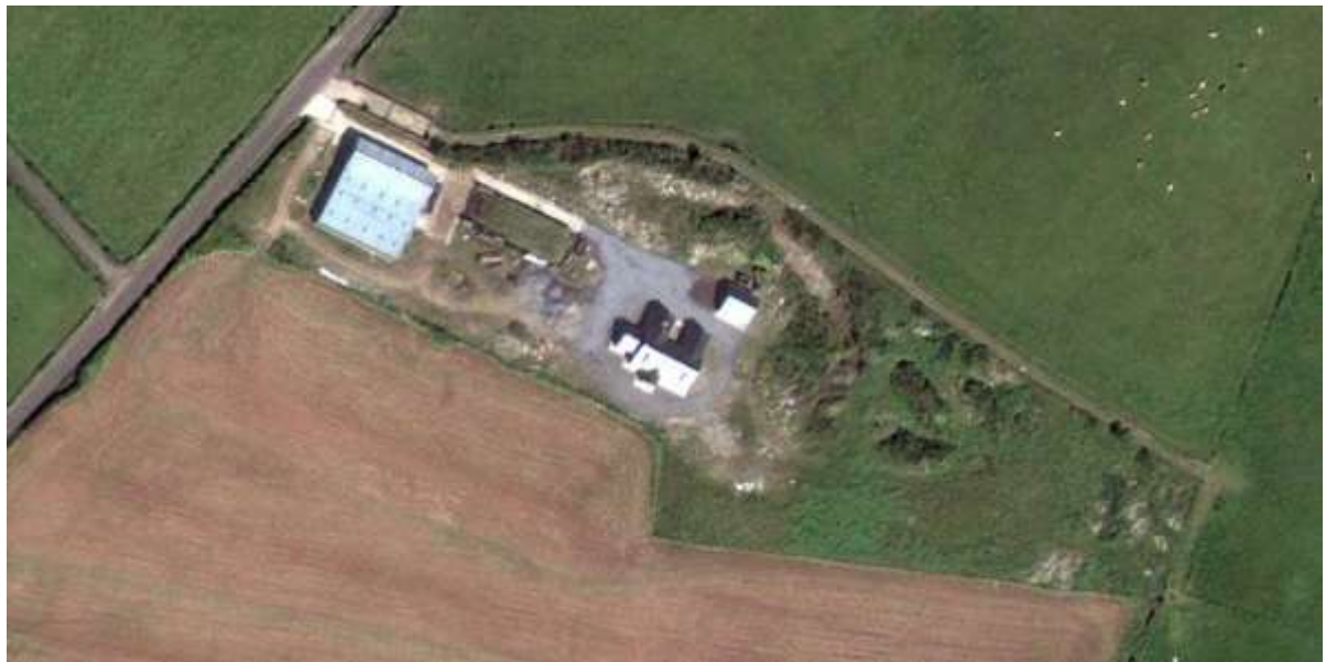
Figure 284 – Site protected in 2009; permission was already granted for development at this site in 2007
