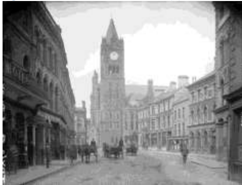
Figure 397 – Foyle Street looking north towards Guildhall (c) NLI
