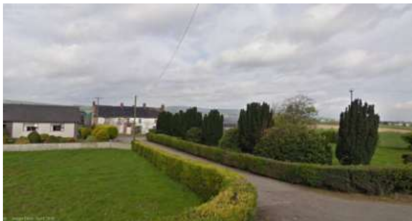
Figure 197 – 18 th century vernacular farmhouse with rare St. Johnston slate roof; structure currently at risk (c) Google
