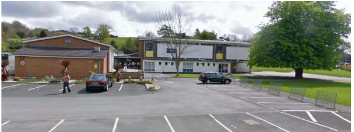
Figure 237 – former Outpatient Clinic, Strabane. Corr & McCormick 1962
