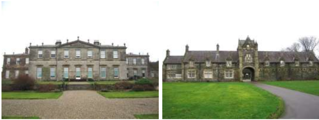
Figure 201 - Baronscourt House and Stables. Source: Natural Stone Database
