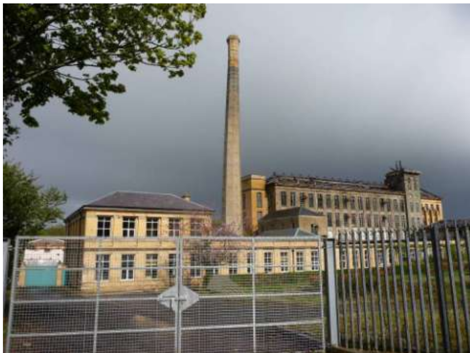
Figure 218 – Herdman's mill after damage by fire, Sion Mills
