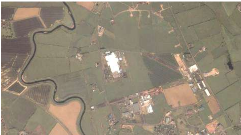
Figure 91 - Aghanloo/Limavady Airfield; aerial view (c) Google
