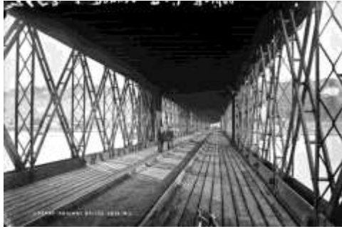
Figure 369 – Craigavon Bridge, lower deck (used for transfer of goods wagons between standard gauge GNR and Northern Counties lines and narrow gauge CDJRC & LL&LS lines ; circa 1890 (c) NLI Lawrence Collection
