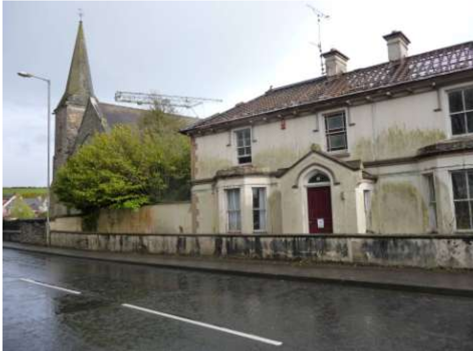
Figure 228 – slates removed from roof of 19 th century house, Newtownstewart
