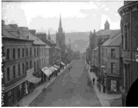
Figure 399 – Carlisle Road looking south towards the bridge (c) NLI
