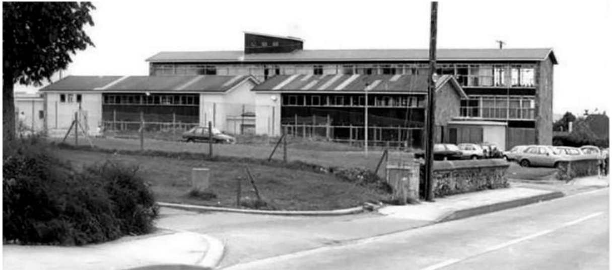
Figure 236 –St. Colman's School , Strabane, Coor & McCormick 1958 (Demolished)
