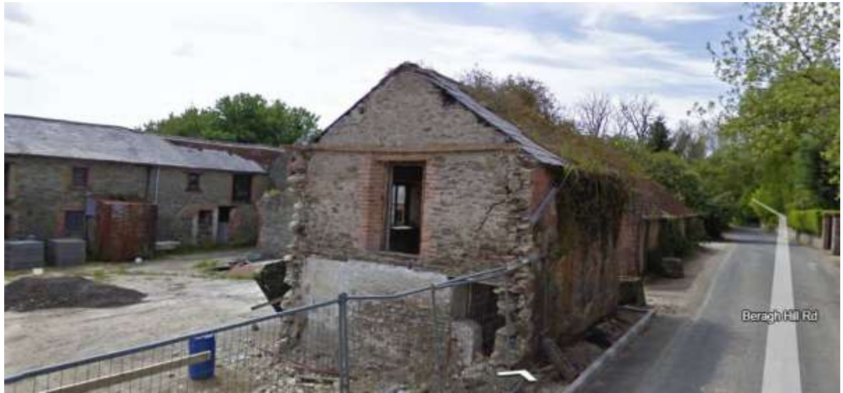
Figure 309 – HB01/27/018 Same buildings from “Streetview” (c) Google
