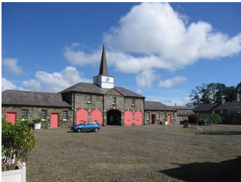
Figure 35: Courtyard Buildings Bellarena Estate. Source: NIEA Natural Stone Database
