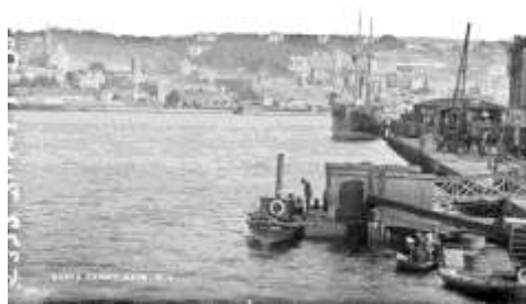
Figure 384 – View of Waterside from city quays (c) NLI
