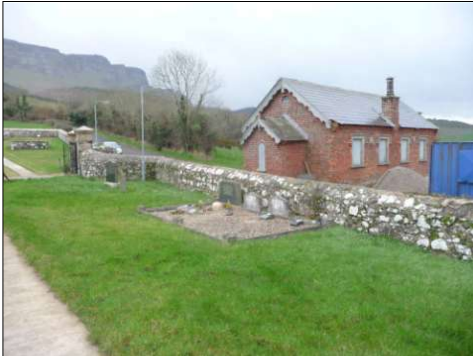
Figure 42: St Cadan's church hall
