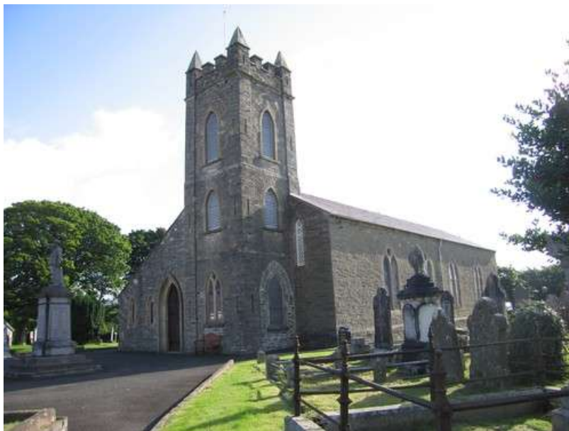
Figure 152 – Glendermott Parish Church. Source: Natural Stone Database
