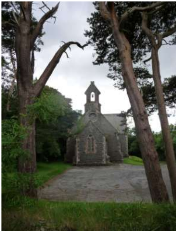
Figure 184 – St Finian's church, Redcastle; designed by Welland & Gillespie
