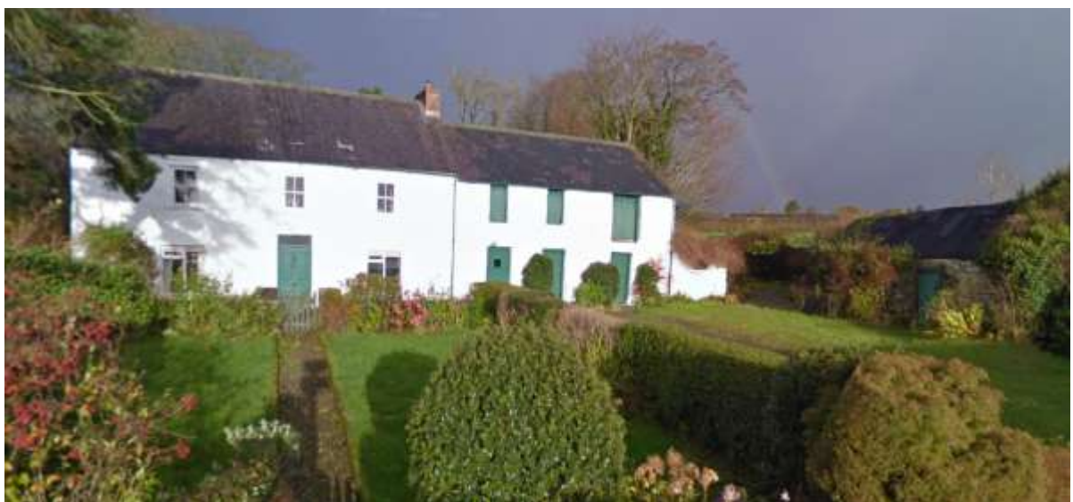
Figure 143 – vernacular house, Eskaveen (c) Google
