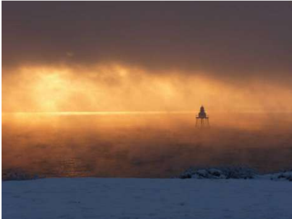
Figure 234 – Moville Light, Mitchell screw-pile lighthouse
