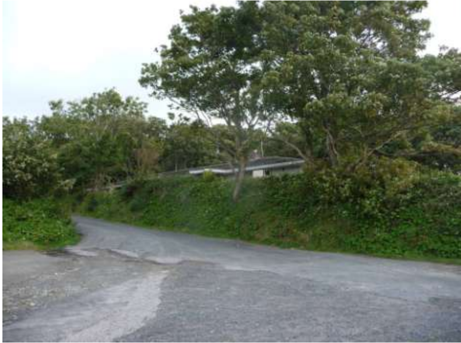
Figure 198 - Liam McCormick designed house, Glenburnie, Moville
