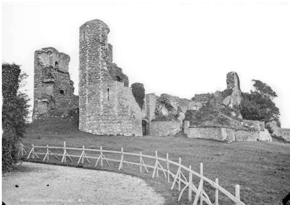
Figure 263 – Northburg/ Greencastle (c)NLI
