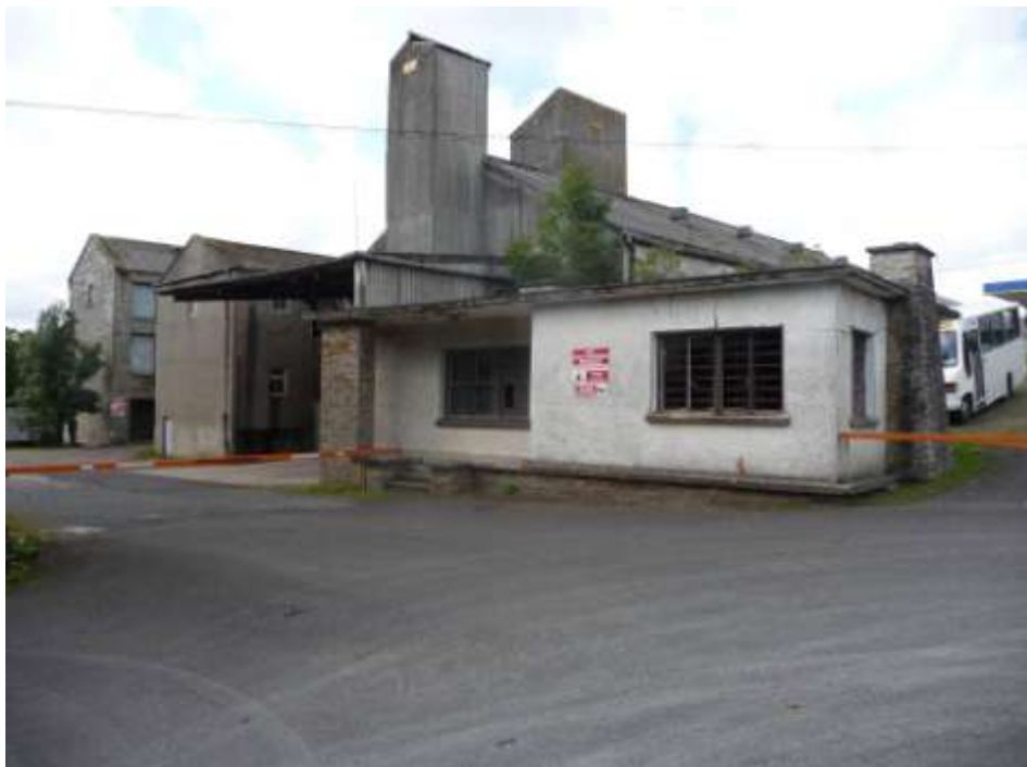
Figure 228 – McCauley's Mill, Moville; gate lodge is Liam McCormicks first commission
