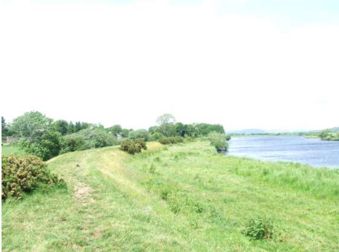
Figure 58 – Foyle flood embankment, Port Hall
