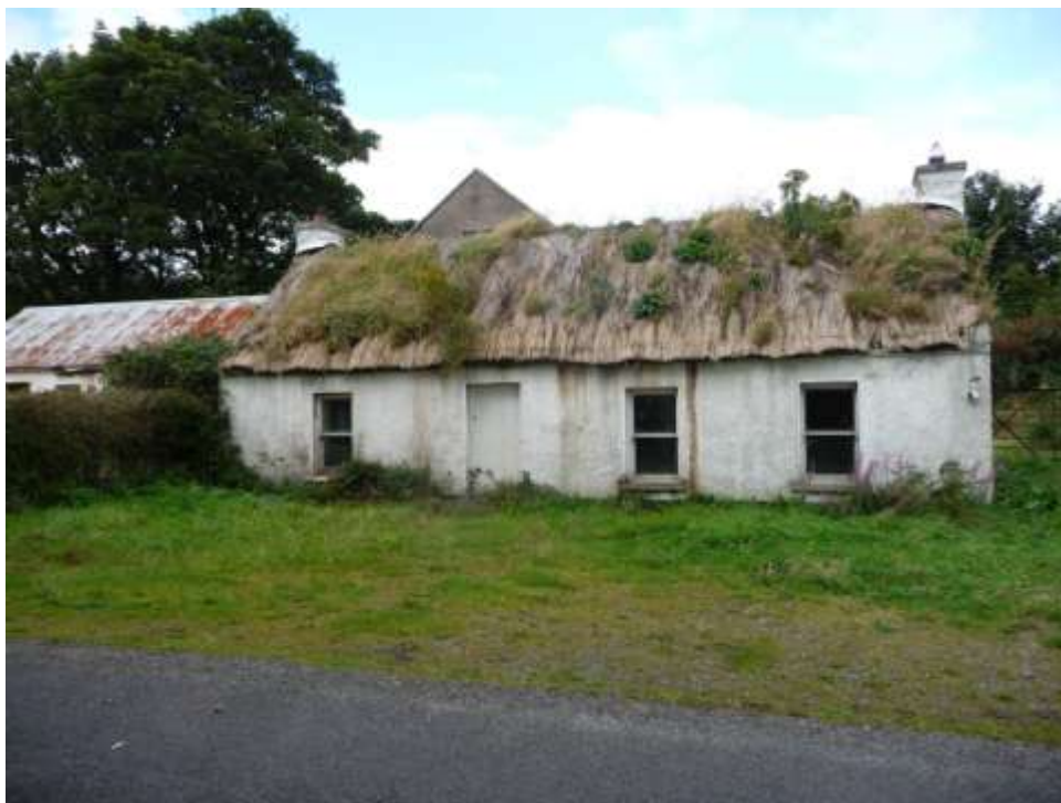
Figure 190 – thatched house, Stroove
