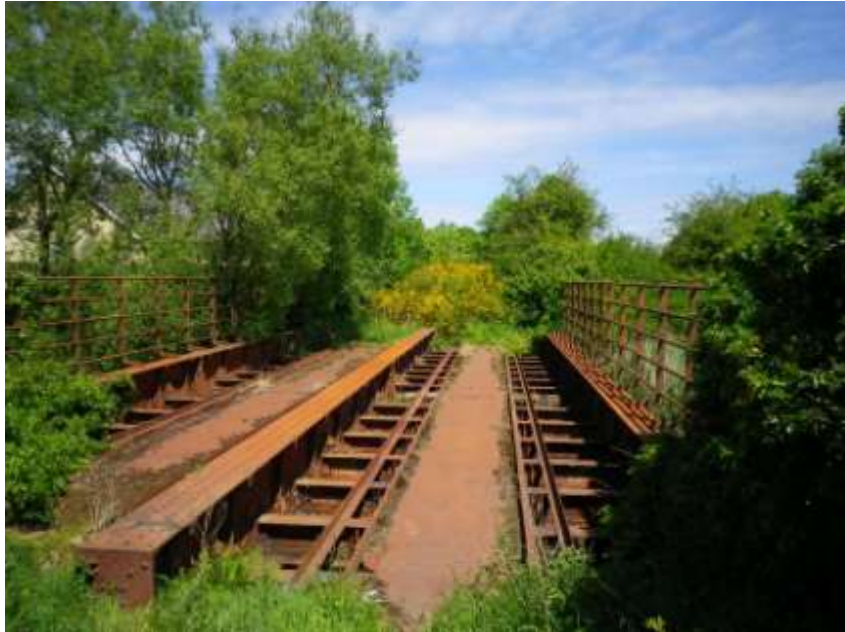
Figure 105– Railway bridge St Johnston
