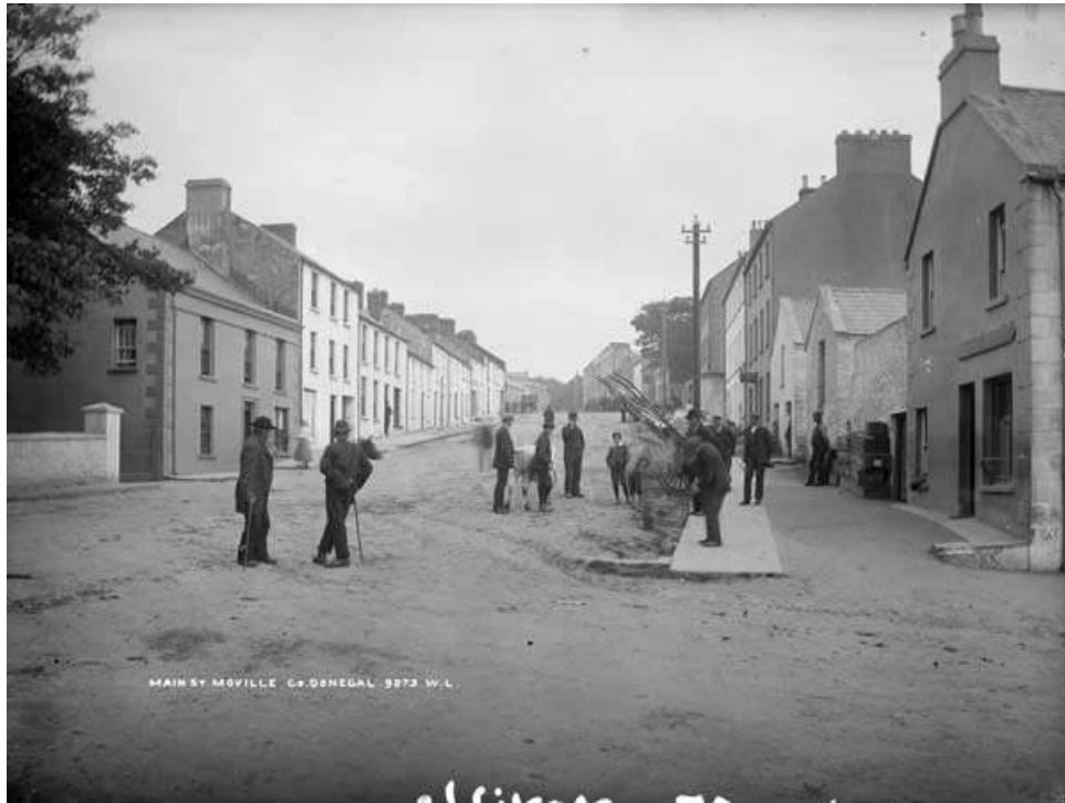
Figure 248 – Lower Main Street Moville (c)NLI
