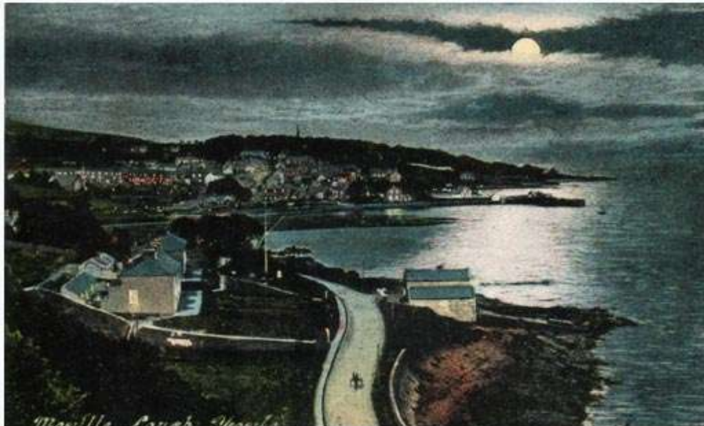
Figure 270 – approach to Moville from Derry (c)NLI
