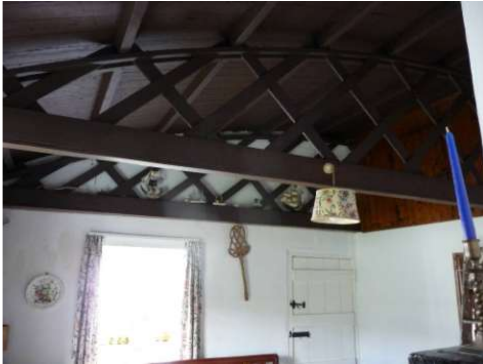
Figure 193 – the “Onion Baskets” Belfast roof structure
