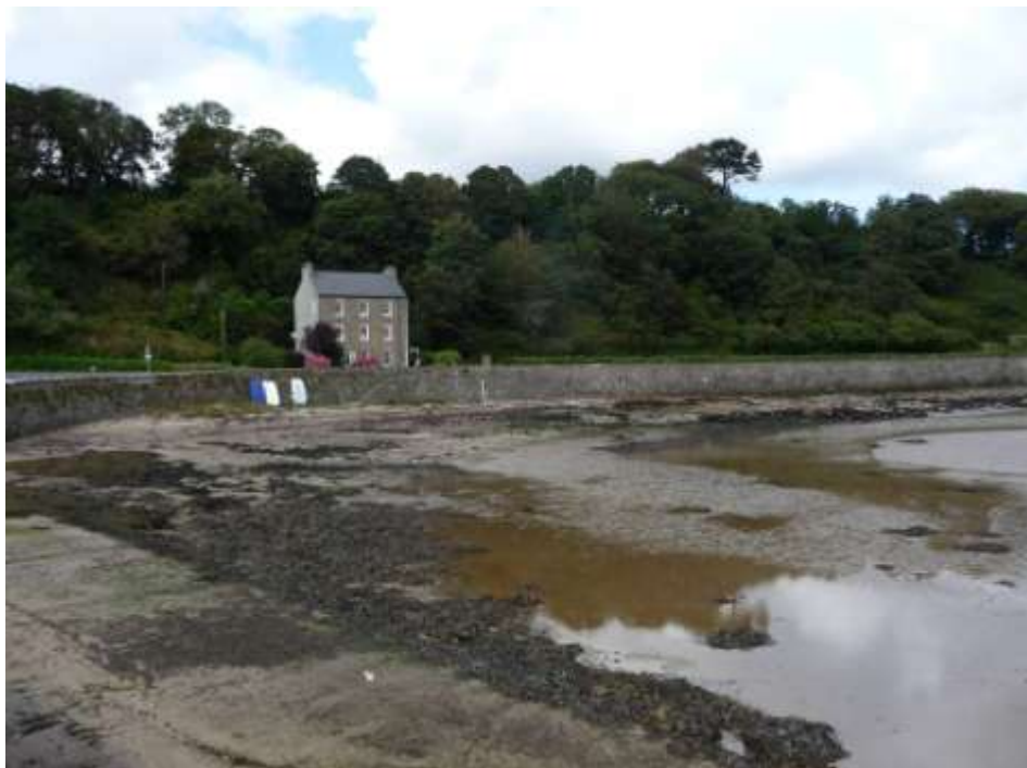
Figure 212 – Carrickarory House, Moville
