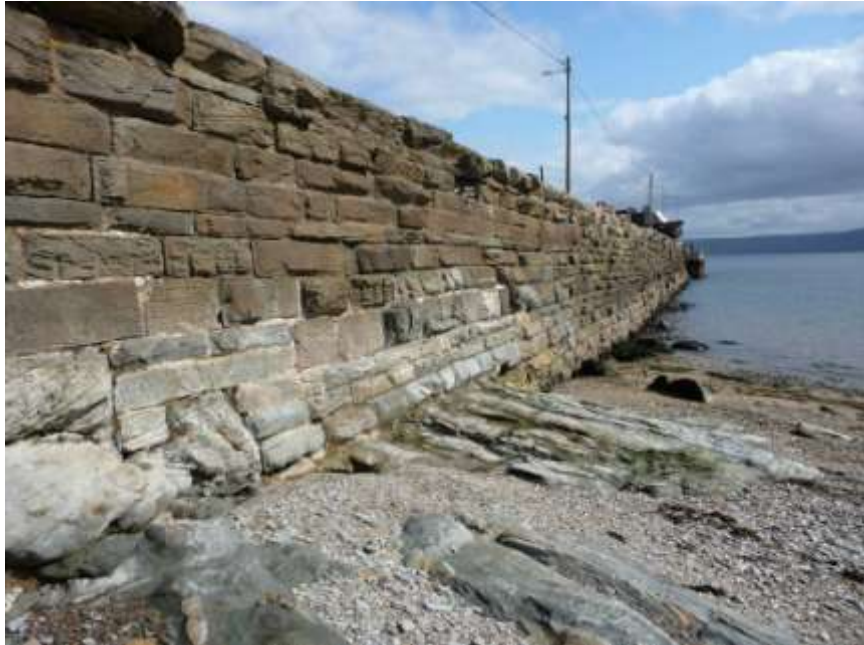
Figure 236 – Carrickarory pier, Merville
