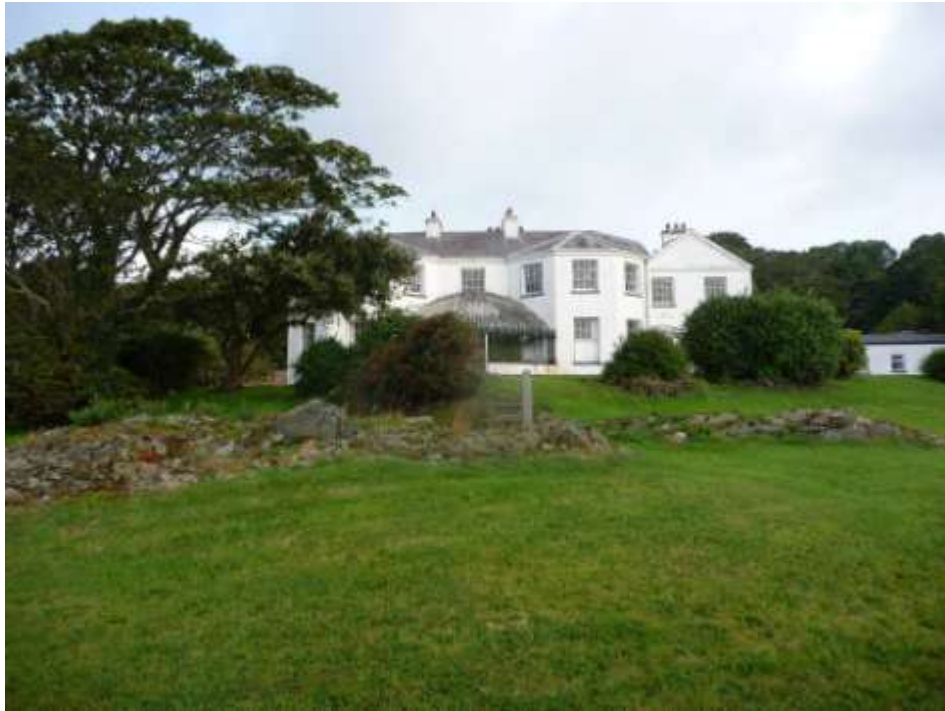
Figure 200 – Carnagarve House, Merville; curvilinear glass house to front attributed to Richard Turner
