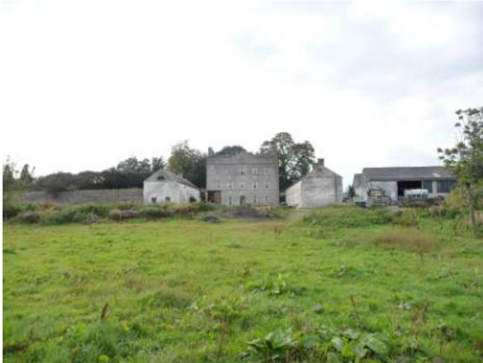
Figure 56 – Port Hall, former Port side
