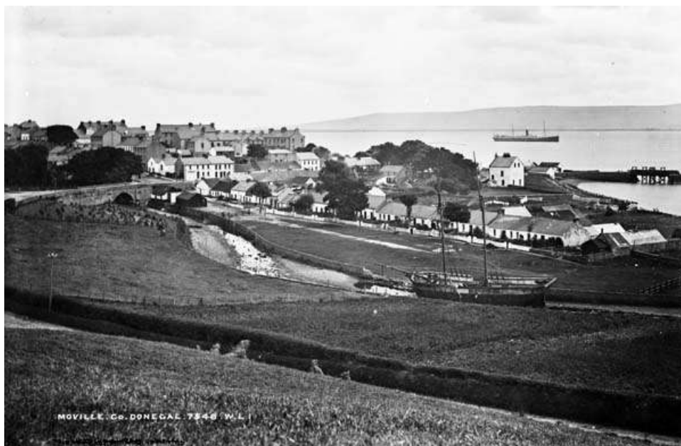
Figure 251 – Approach to Moville from Derry (c)NLI
