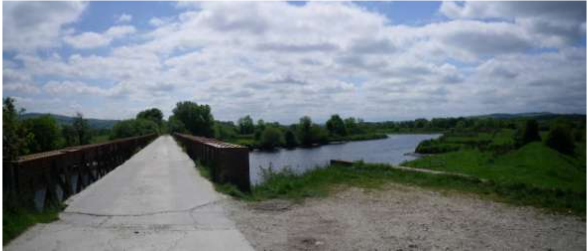
Figure 64 – Corkan Isle trestle bridge
