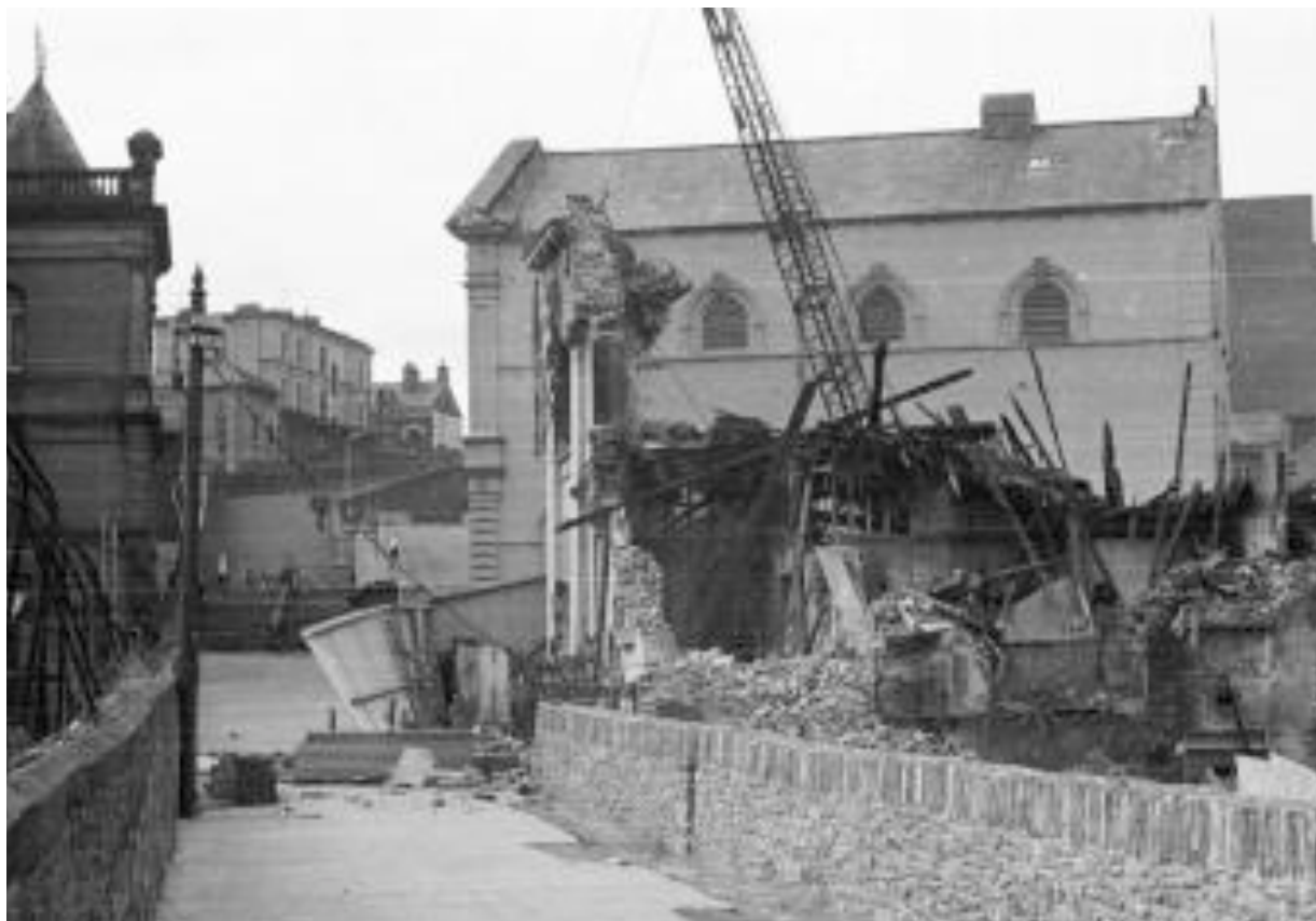
Demolition of buildings along East Wall, circa 1970
