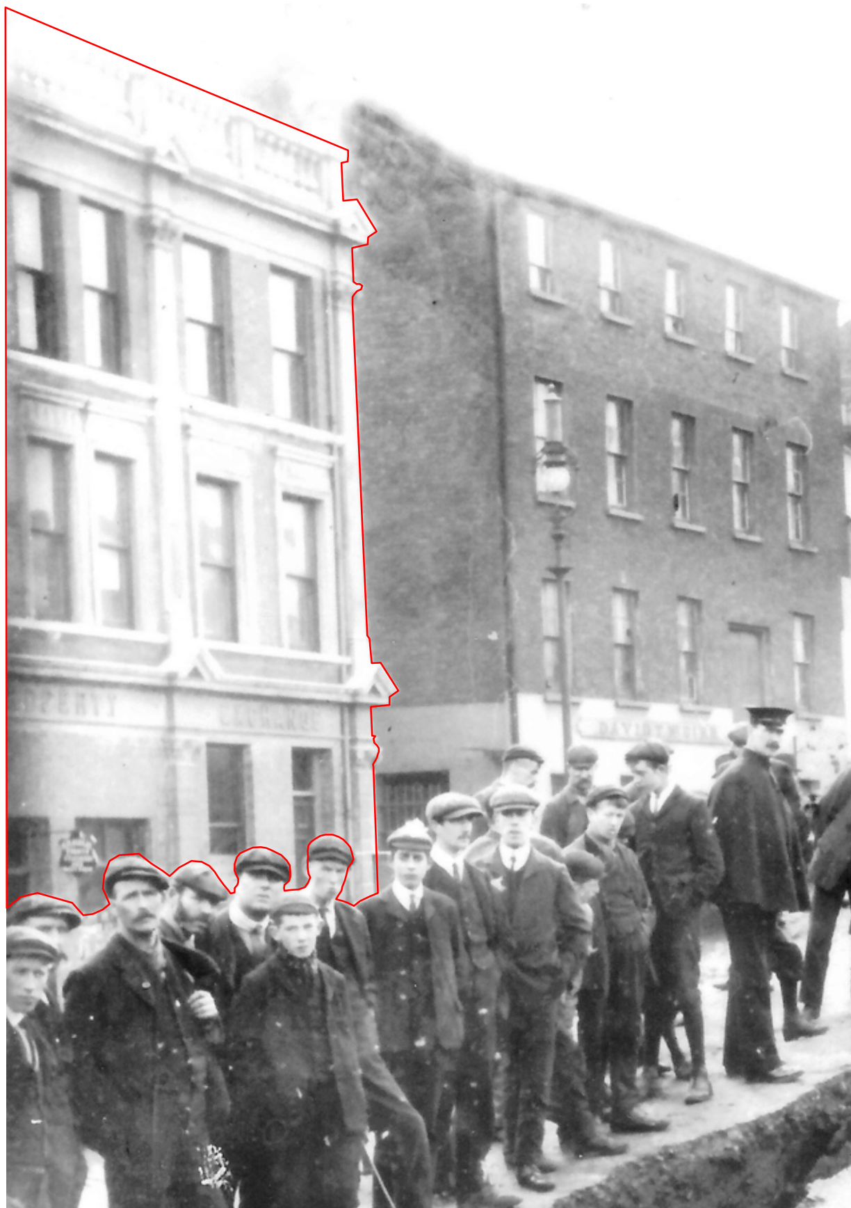
Collapse of the City Walls, Lower Magazine St, circa 1910. Photograph shows Magazine St elevation of Nos. 12-14 Castle St (CS5, right within outline) and No.11 Magazine St (LM6, left within outline).
