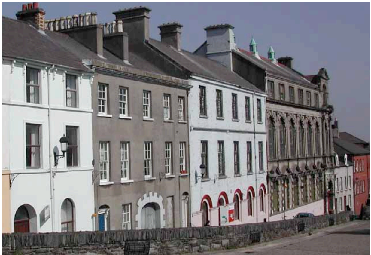
The Playhouse, 5-7 Artillery Street, prior to restoration. Photograph circa 2004.
