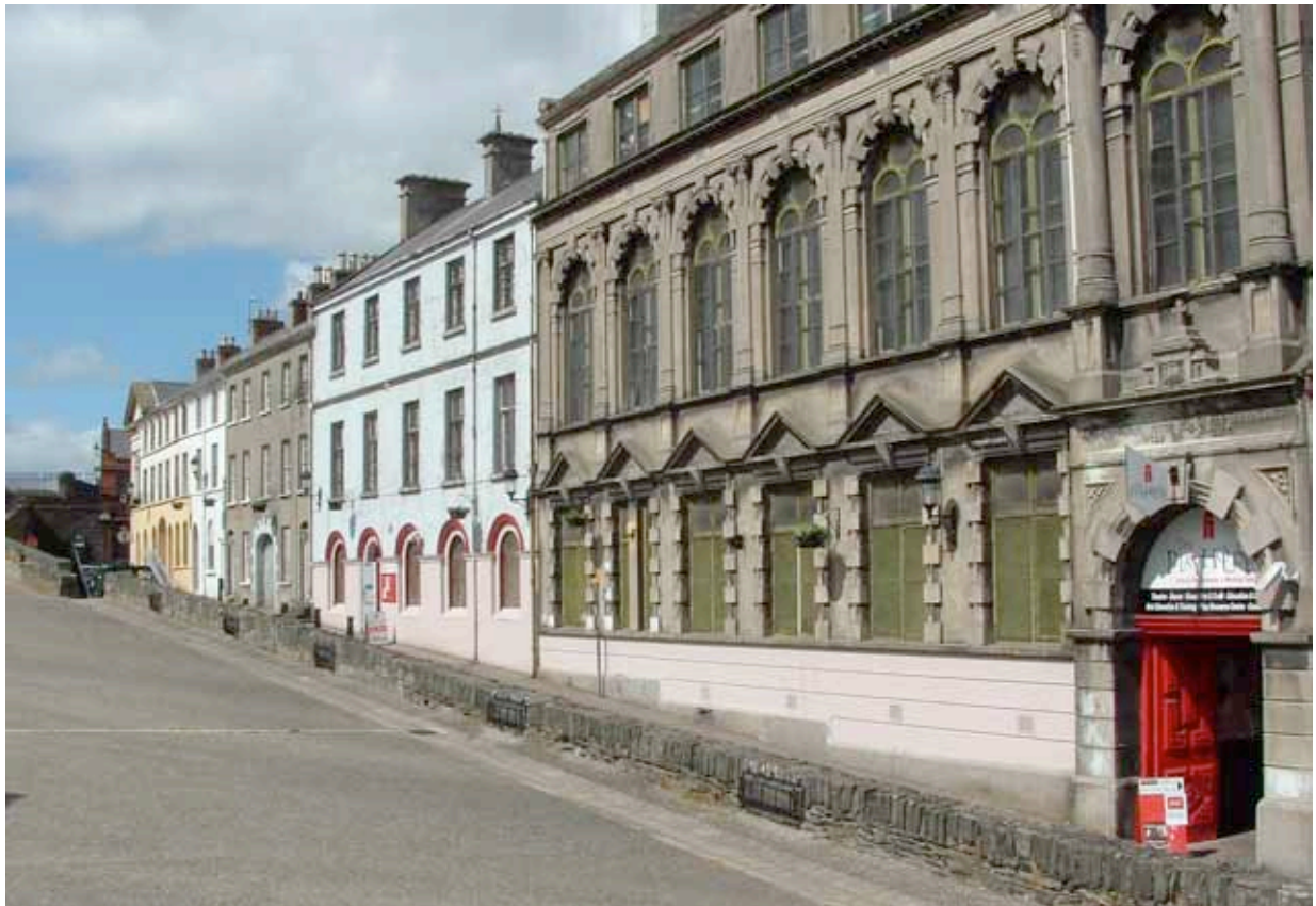
The Playhouse, 5-7 Artillery Street, prior to restoration. Photograph circa 2004.
